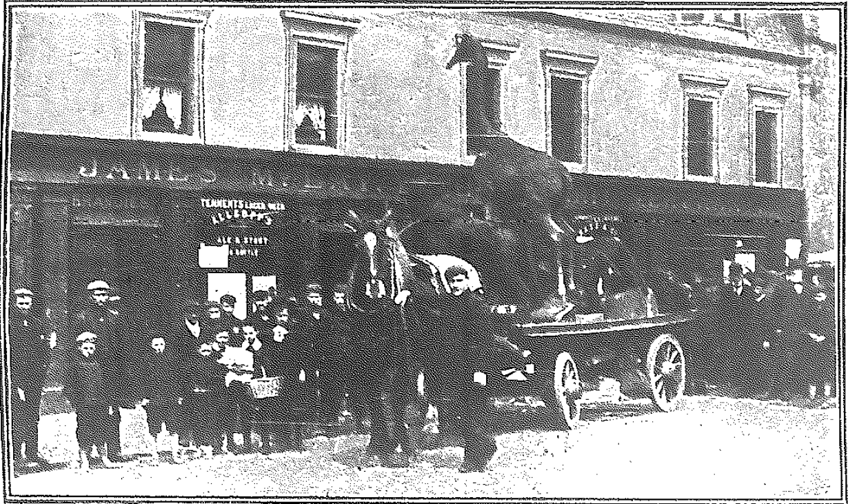
The Paisley Central Hall Site: Clearing out the Museum Bar
